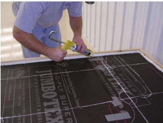
Figure 16: Sealing P2 edge
