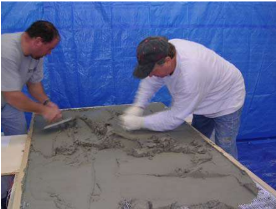
Figure 36: Mortar application
