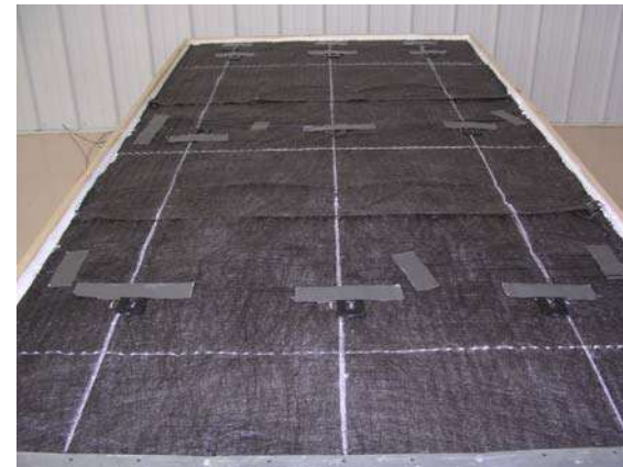
Figure 23: Sure Cavity layer completed
