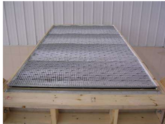
Figure 27: Metal Lath Layer completed
