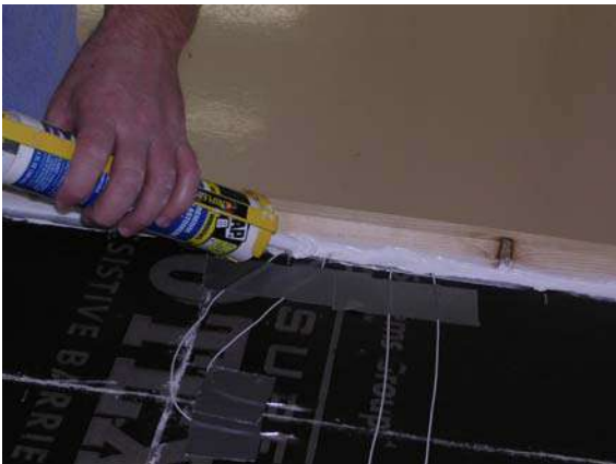
Figure 10: Sealing paper edge
