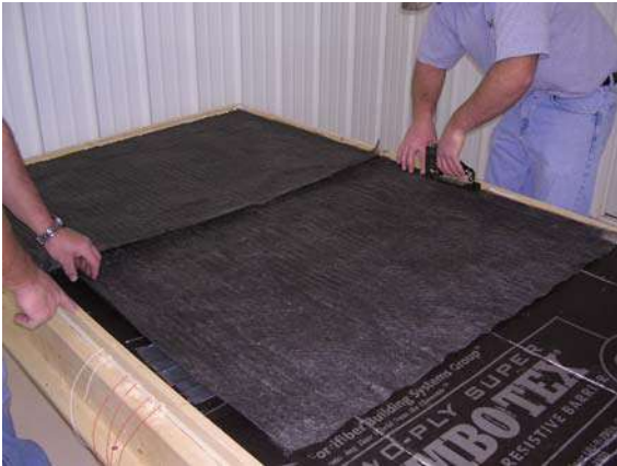
Figure 18: Sure Cavity layer placement
