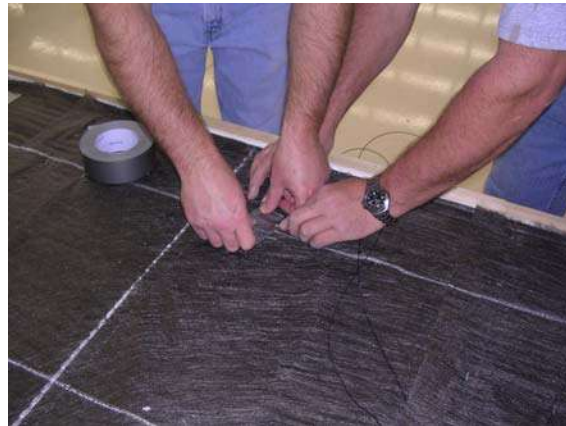
Figure 21: Securing sensor wires
