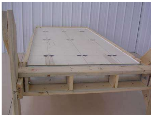
Figure 5: Plywood Layer completed.
