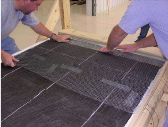
Figures 24: Installation of metal lath, Panel A
