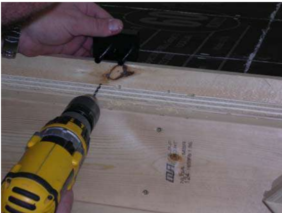
Figure 8: Sensor wire guide hole placement
