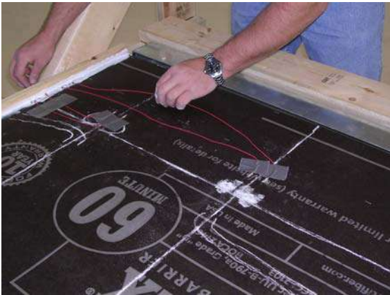
Figure 14: Affixing sensor wires
