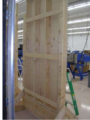
Figure 2: Rear view of frame construction
