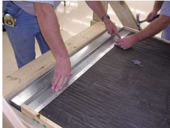
Figure 19: Weep screed installation
