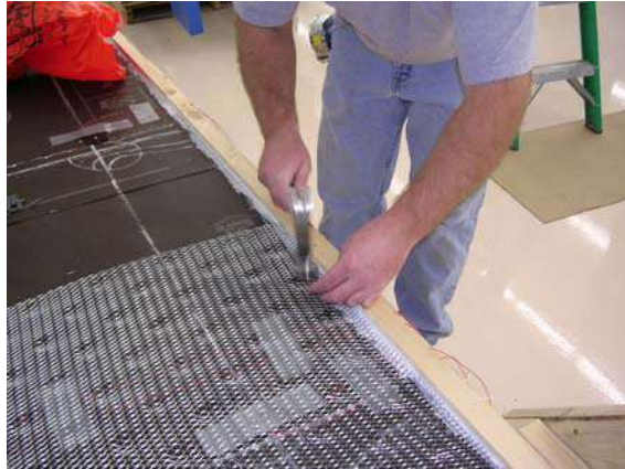
Figure 25: Installation of metal lath, Panel B
