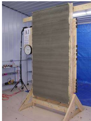
Figure 39: Scratch coat completed
