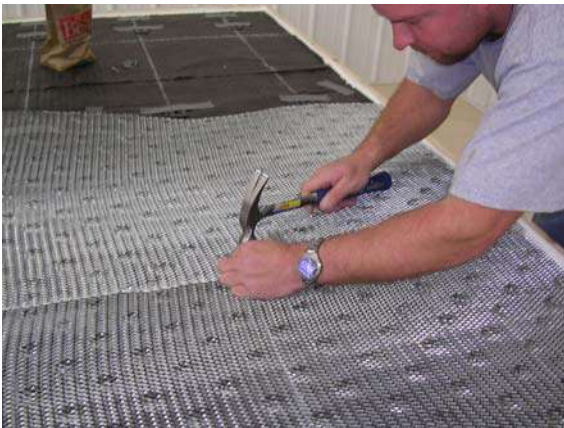
Figure 26: Installation of metal lath
