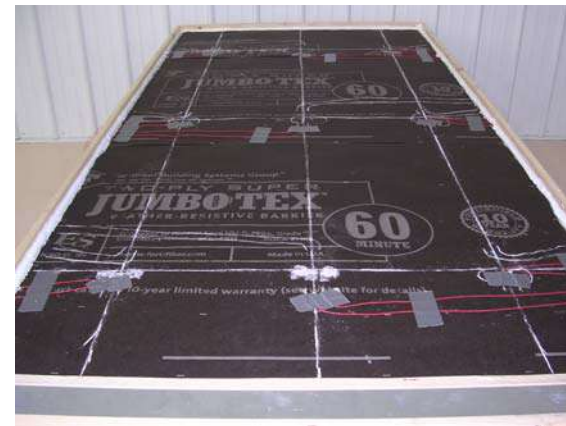
Figure 17: Paper Layer 2 completed
