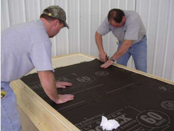
Figure 6: Construction paper placement
