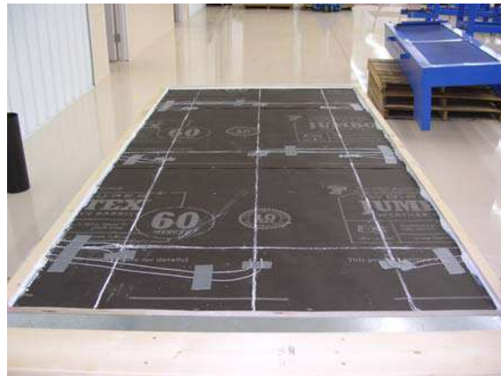
Figure 11: Paper Layer 1 completed
