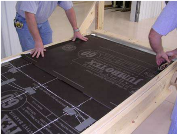
Figure 12: Installation of second paper layer
