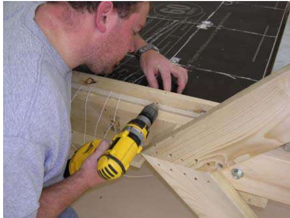
Figure 13: Drilling sensor wire guide holes
