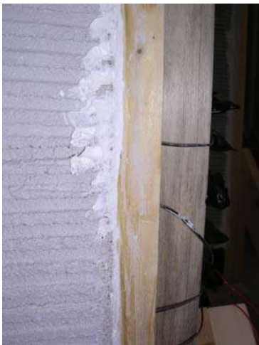
Figure 38: Sealed mortar edge
