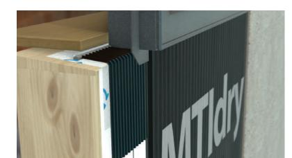
Corrugations create a gap for drainage in window sub sill
