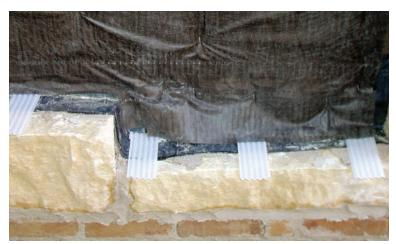
Wall Opening Weeps with Sure Cavity on natural stone
