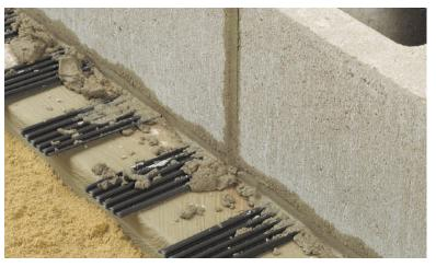
Vent Mat creates multiple weep tunnels in each block core
