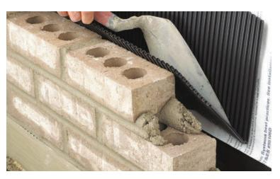
Trash Mortar Diverter is placed in the cavity on brick ties
