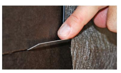
Moisture Diverter directs moisture from the rainscreen drainage plane away from windows & wall openings
