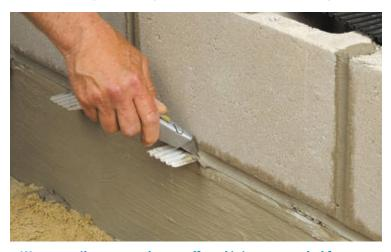
Weeps easily score and snap off, and joints are tooled for a finished appearance
